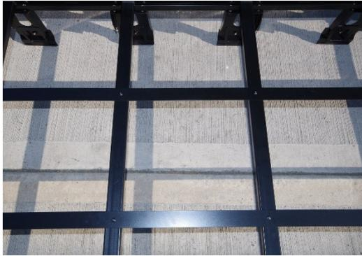
7. Using a pop rivet gun, insert one rivet into every crossbar intersection.
