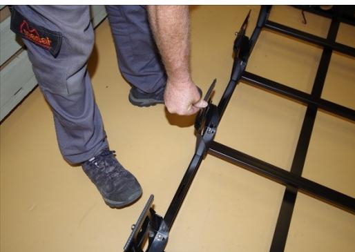
5. Push a protective rubber pad onto each of the legs and use the foam material provided with the packaging to line the underside of the brackets.
