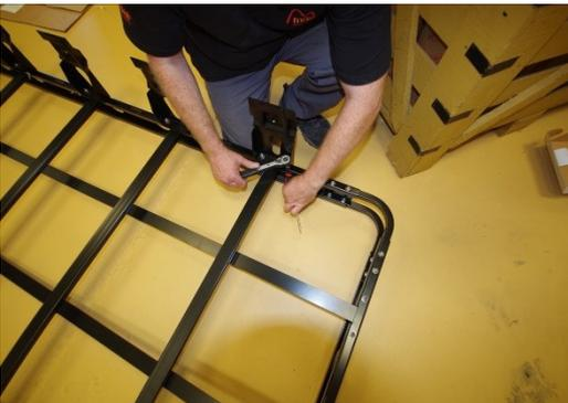
3. Assemble the leg brackets, crossbars and side panels as shown. Usually, the legs will sit flush with the side panel, but the oblong hole on the leg bracket allows you to adjust the position if necessary.
